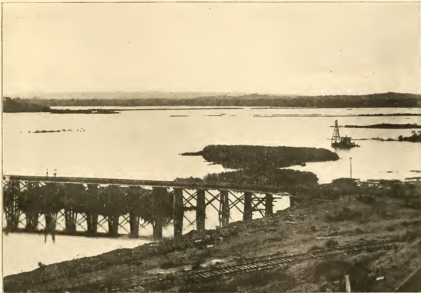
GATUN LAKE. FLOATING ISLANDS MASSED AGAINST TRESTLE
